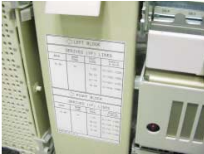
Figure 23. Example of Original (Unmarked) Protector Block Label
