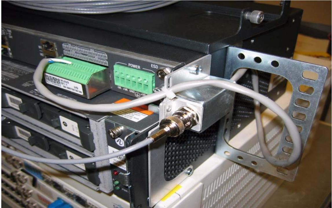
**Figure 3-21** Left side E1 input timing cable mounting position
