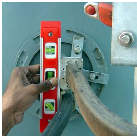
Figure 5-1. Checking Feedhead Flange with a Spirit Level
