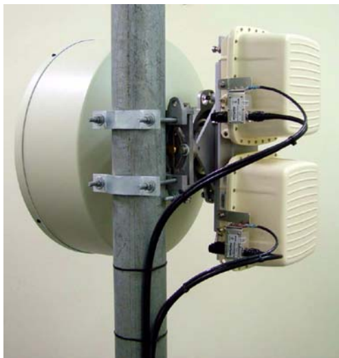
Figure 2-12. Coupler Installation with ODUs
